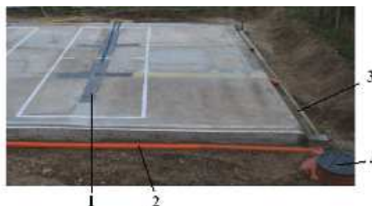
Fig. 3 - Drainage and collection system
