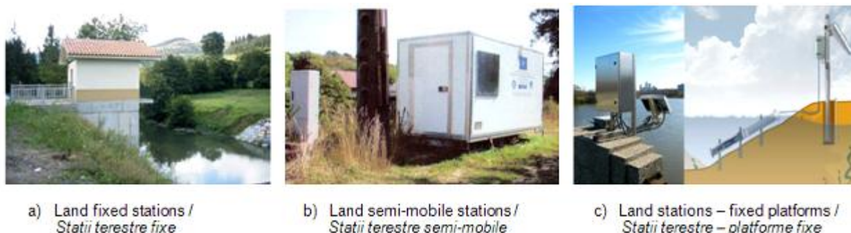
Fig. 3 - Land stations for monitoring of rivers' water quality [6, 7] / Statii terestre de monitorizare a calitatii apei râurilor (a, b - www.hach-lange.ro ; c - www.nexsens.com )
