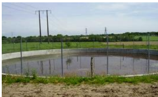
Fig. 3. - Uncovered, closed tank, for fluid dejections (slurry) collection, according to EU regulations, [1]
