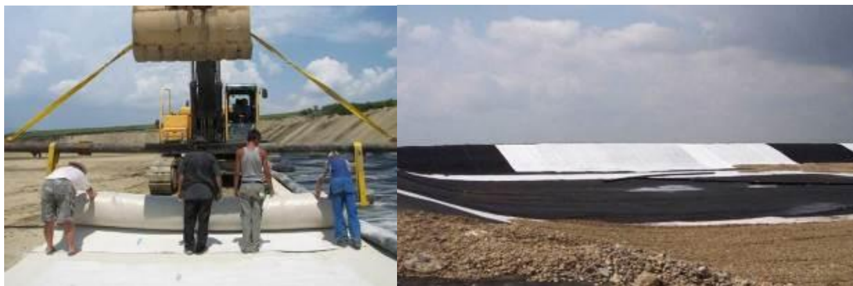
Fig.1 – Examples of geomembrane and protection geotextile utilisation in the construction of waste landfills
