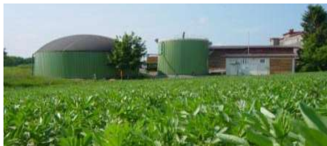
Fig. 6 - Vertical digester in Germany, for the processing of manure from swine and poultry farms and silage ( Al Seadi, 2001 )
