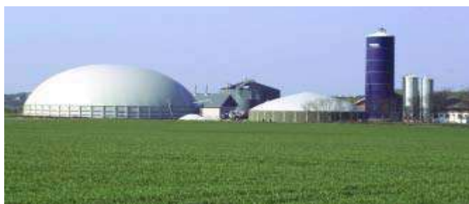
Fig. 5 - Image of a Danish farmer-level biogas plant, that co-digests animal waste and energy crops ( Al Seadi, 2001 )
