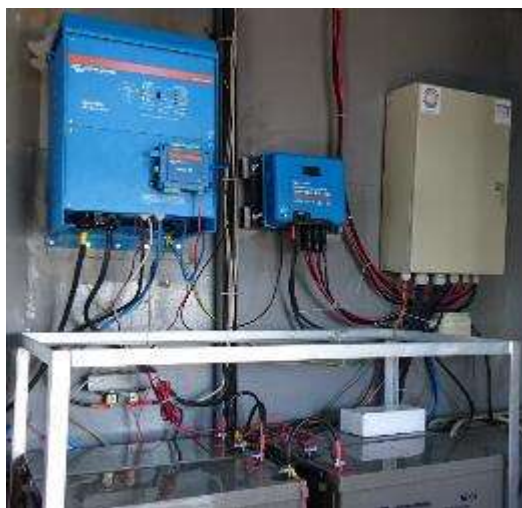
Fig. 3 - Components of the photovoltaic system (accumulators, solar charger and inverter with switching unit)
