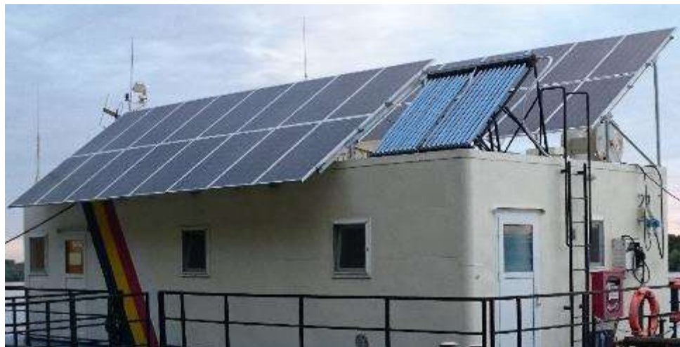
Fig. 1 - The components of the system installed on the roof of the pontoon
