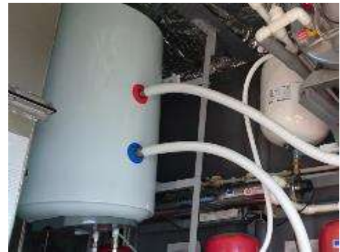
Fig. 8 - Boiler and solar pipes
