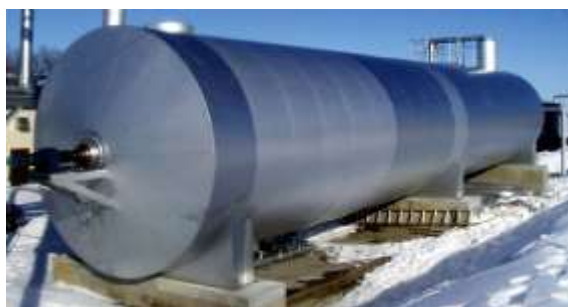
Fig. 3 - Horizontal digester, built in Denmark ( Nordisk Folkecenter, 2001 )
