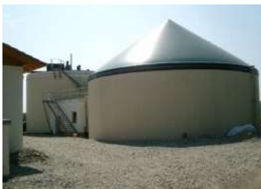
Fig. 7 - Vertical digester from Germany, built in 2005 for the digestion of biomass from energy crops (Al Seadi, 2001; Hanxi et al, 2018)
